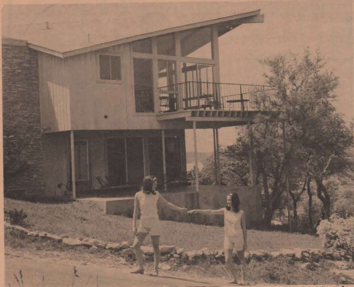
HILLSIDE HOME — The three-level home of Mr. and Mrs. Charles R. Rose in Canyon Lake Village was built by Helms Lumber Co. with a breathtaking view across the nine-mile length of the reservoir. The architect for Helms slept
