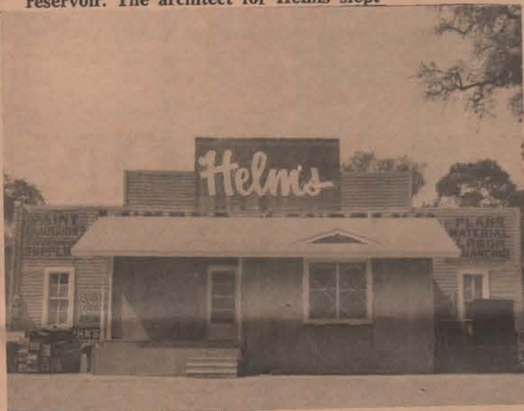
SATTLER LANDMARK — The Helms Lumber Co. building at Sattler was once Valhalla Hall, scene of lively dancing for generations. The company prides itself on complete "turnkey" work, from planning to finish, even to carpeting on the floors. In Sattler five years and in the building business 25 years, Helms is also established in Wharton and New Braunfels and soon will open a sales office in Startzville.
