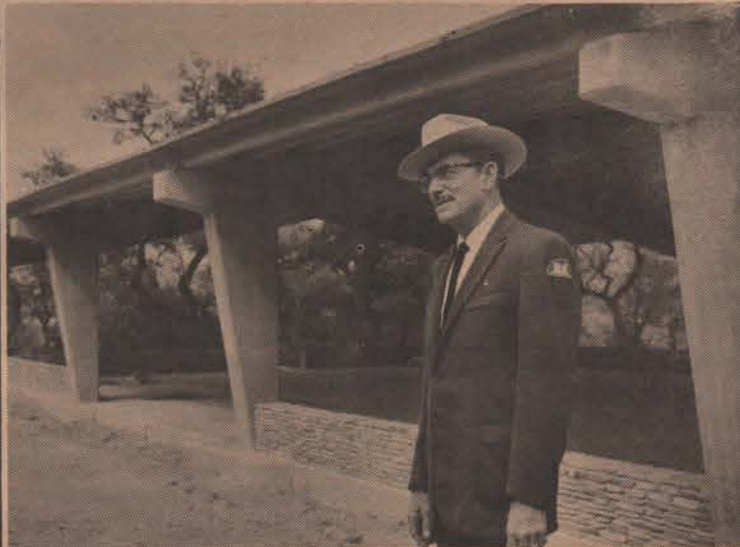
PROJECT ENGINEER — W. F. Humphreys, above, is the project engineer supervising operation and maintenance of the new 8,240-acre Canyon Reservoir for the US Army Corps of Engineers. He is shown at a Canyon Model Park group picnic shelter on the north side of the lake.
