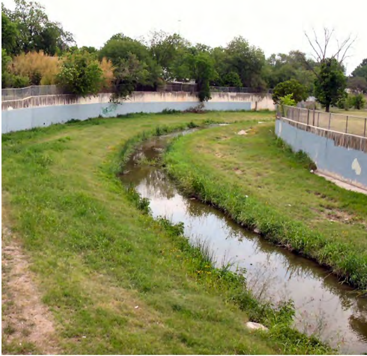
Retaining walls at Martínez Creek
