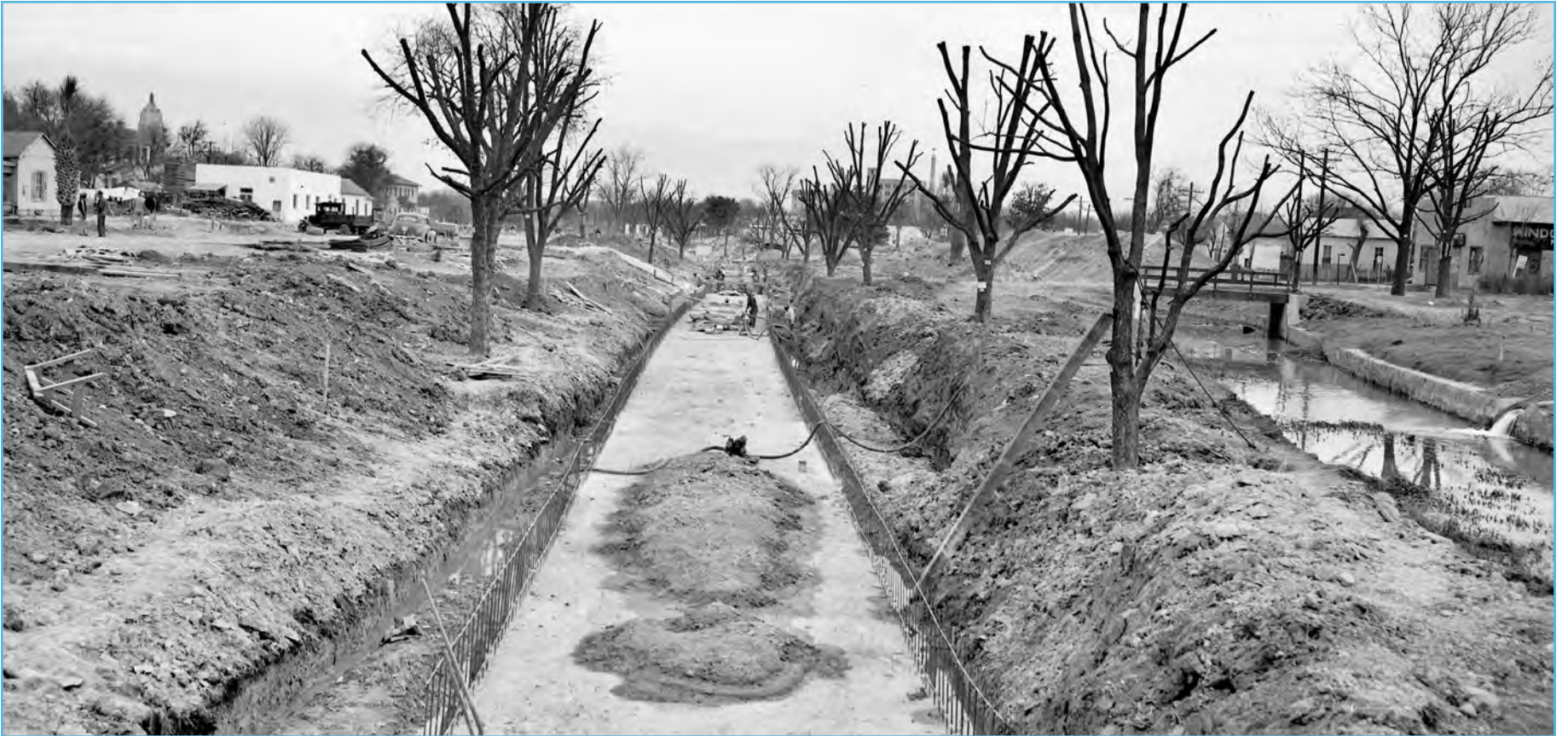
Channel construction for San Pedro Creek in the early 20th century
