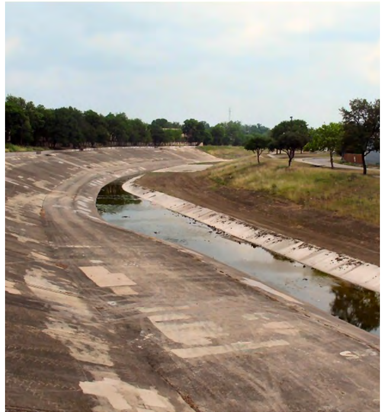
Concrete channel at Apache Creek
