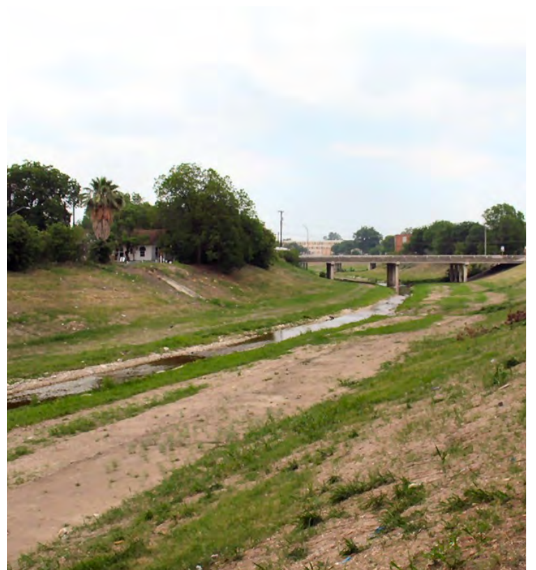
Trapezoidal channel at Alazán Creek
