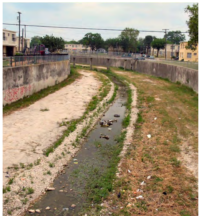
Concrete retaining walls at Alazán Creek
