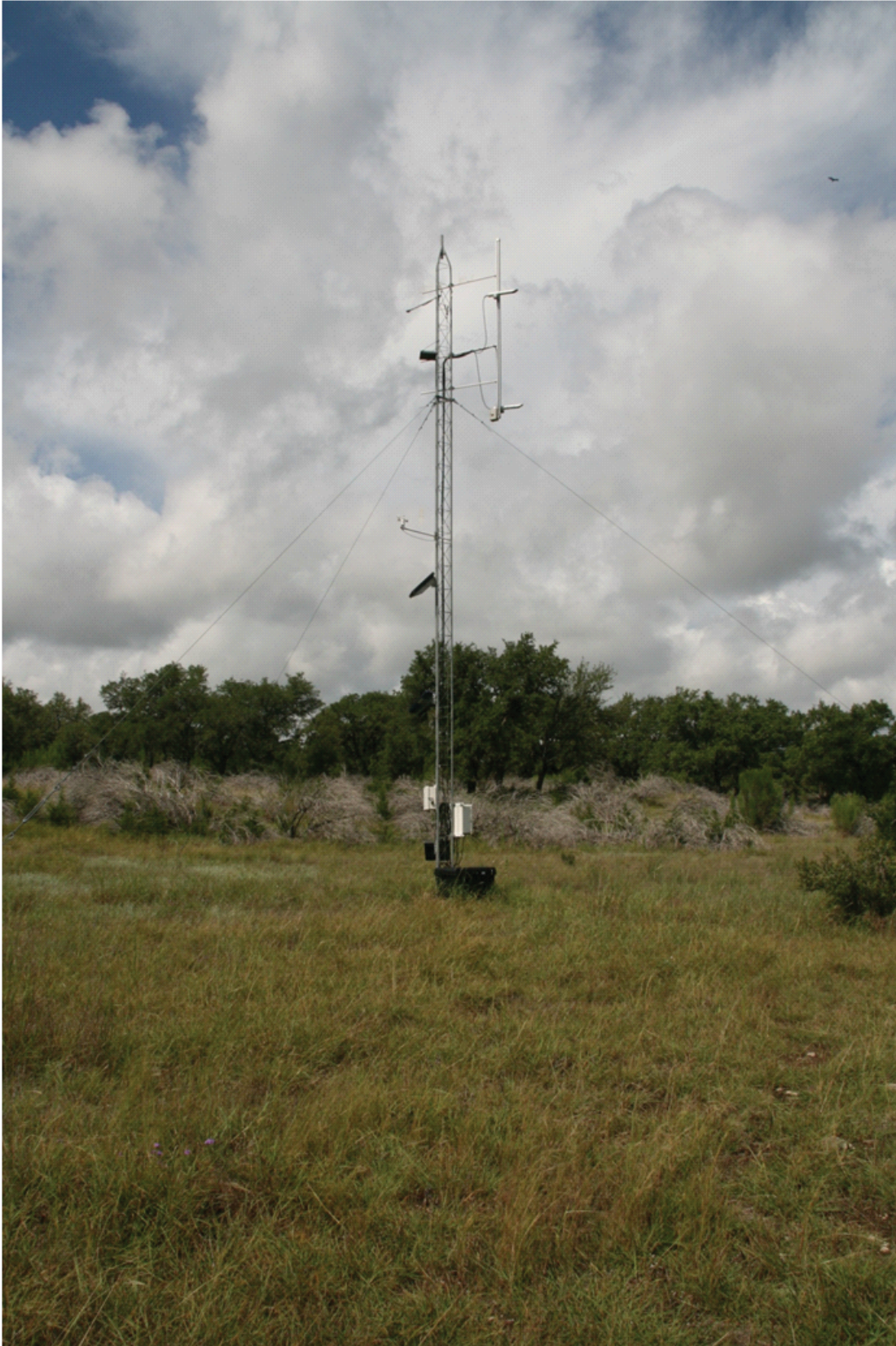
Figure 5. Evapotranspiration station in the treatment watershed at site TWS ET (U.S. Geological Survey station 295102098283200 Honey Creek treatment evapotranspiration near Spring Branch, Texas), Honey Creek State Natural Area, Comal County, Tex., July 23, 2010.
