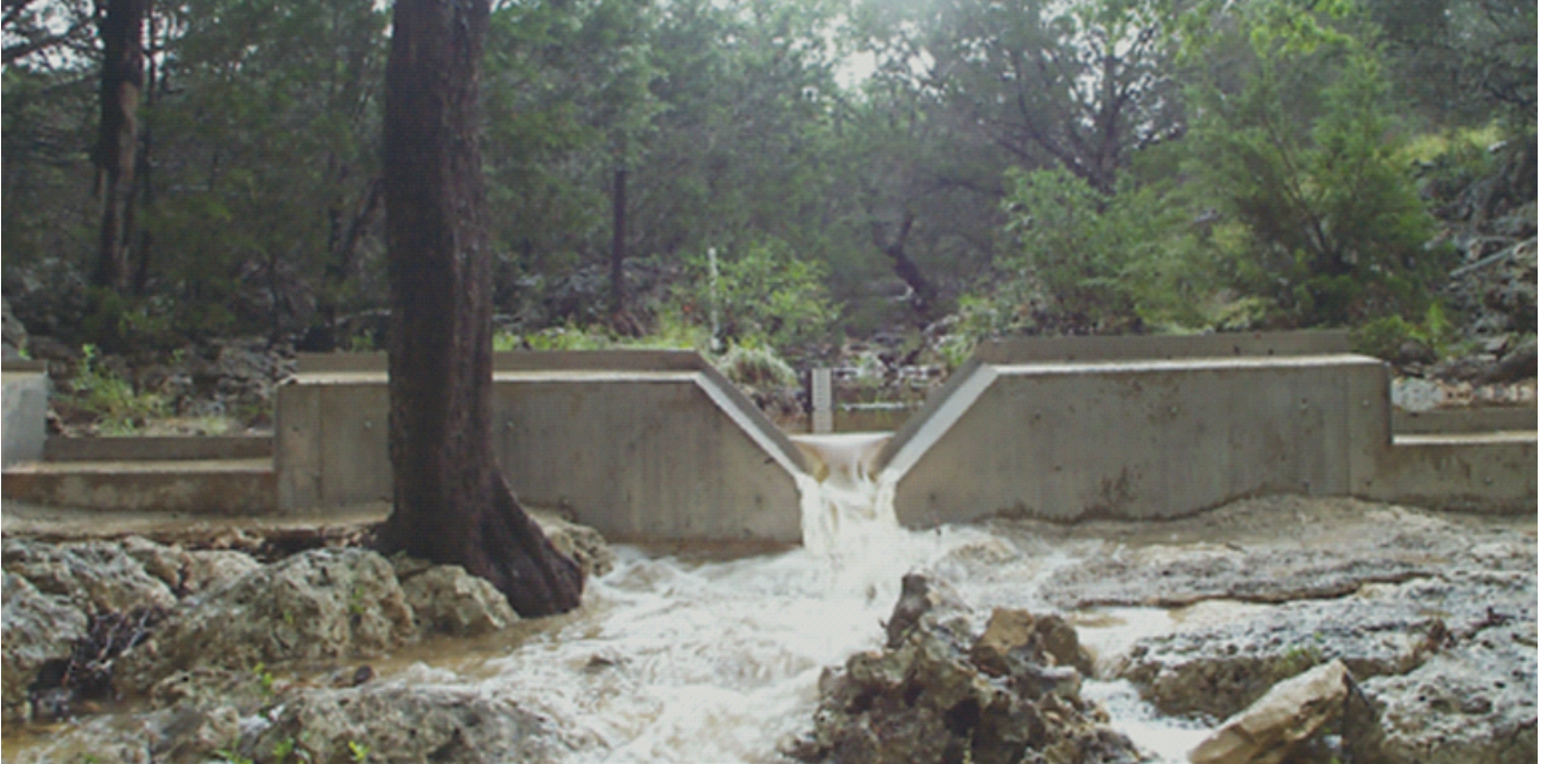
Figure 3. Example of streamflow channel and weir in the treatment watershed at site 2T (U.S. Geological Survey station 08167353 Unnamed tributary of Honey Creek site 2T near Spring Branch, Texas), Honey Creek State Natural Area, Comal County, Tex., June 28, 2004.
